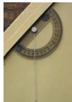
Protractor and plumb line gives the angle of the extractor. Photo by Dr Chris Coulson.
